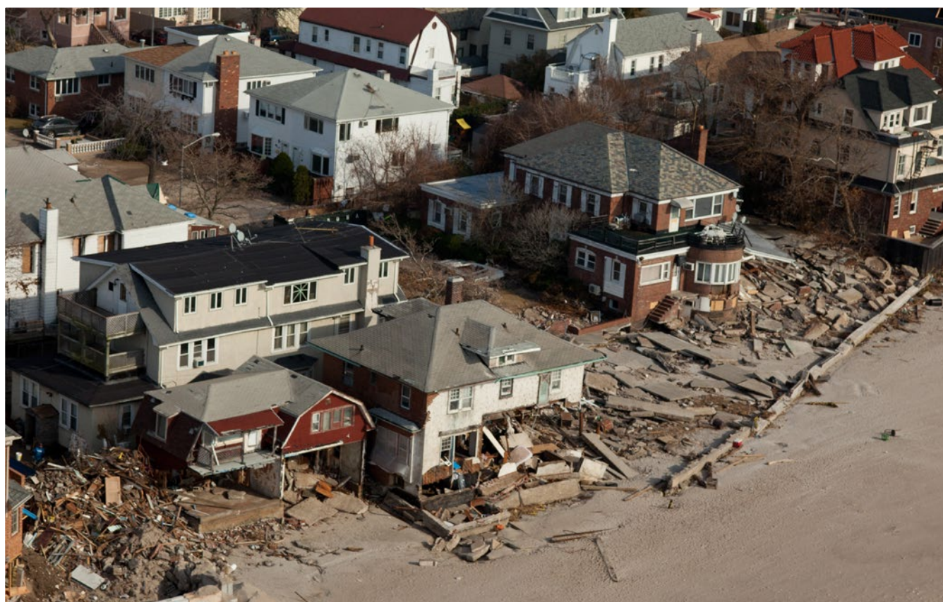
Coney Island, N.Y., Nov. 12, 2012—Aerial view of a Coney Island home moved off of its foundation by Hurricane Sandy. The waves and surge damaged and destroyed thousands of homes on the Eastern coast.
